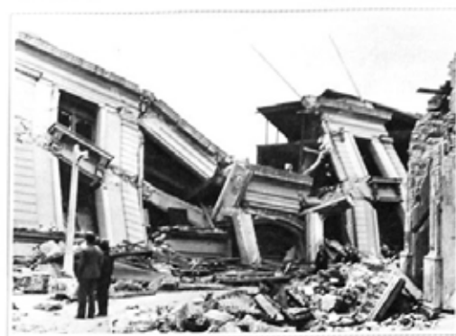
EARTHQUAKE HAVOC IN CHILE: THE FACADE OF THE OFFICE BUILDING OF MESSRS. WILLIAMSON, HARPOUT AND CO., A LARGE FIRM IN CONCEPCION, BROKEN INTO SECTIONS.
